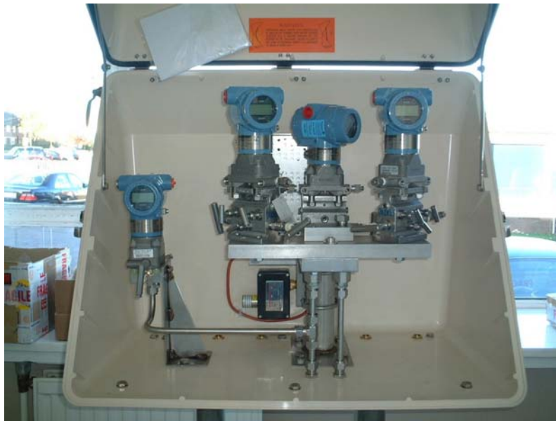
Figure 5: View of enclosure for three differential-pressure transmitters and one static-pressure transmitter (Courtesy of PCD)
